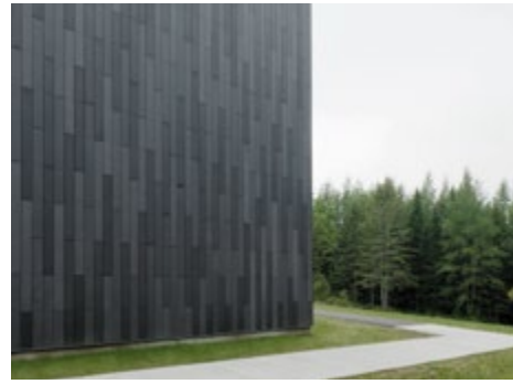
öko skin 147 mm, anthracite, vertical installation (1/3 shifted), screwed on aluminium substructure
