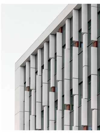
To secure non-visible fastening, an intelligent system with integrated fastening anchors was developed. Weather-proof pre-assembly in the factory guarantees a high standard of quality and rapid assembly on-site. The elements are simply hung into place and finely-adjusted into position.
