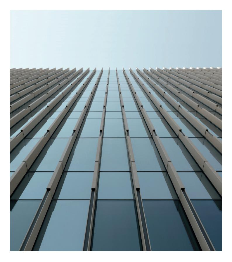
**formparts**folded glassfibre reinforced concrete panels for facades
